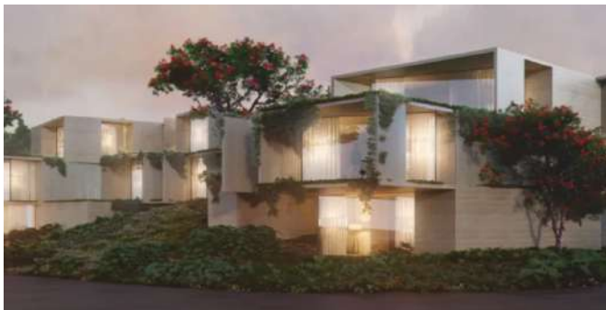
Figure 13,14: Project reference of Partanna's carbon-negative concrete homes developed in the Bahamas. These structures use desalination brine and natural binders, actively sequestering CO 2 during curing and demonstrating a scalable model for climate-resilient, low-carbon housing.
