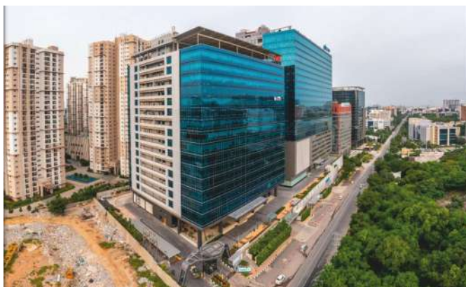
Image 1: Phoenix Aquila, Hyderabad (2 Basements + Ground Floor + 7 Stilt Floors + 16 Upper Floors.); Height:106 mtr; Area Apx: 1.3 Million sft ; Project Status: Structure Completed.
